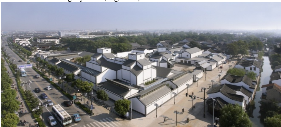
Fig. 4 Aerial View of the New Suzhou Museum Picture Source: Internet
