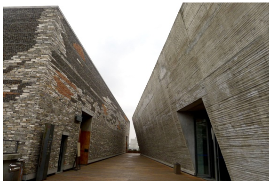
Fig. 9 "Bamboo Strip Formwork Concrete" Picture Source: Internet
